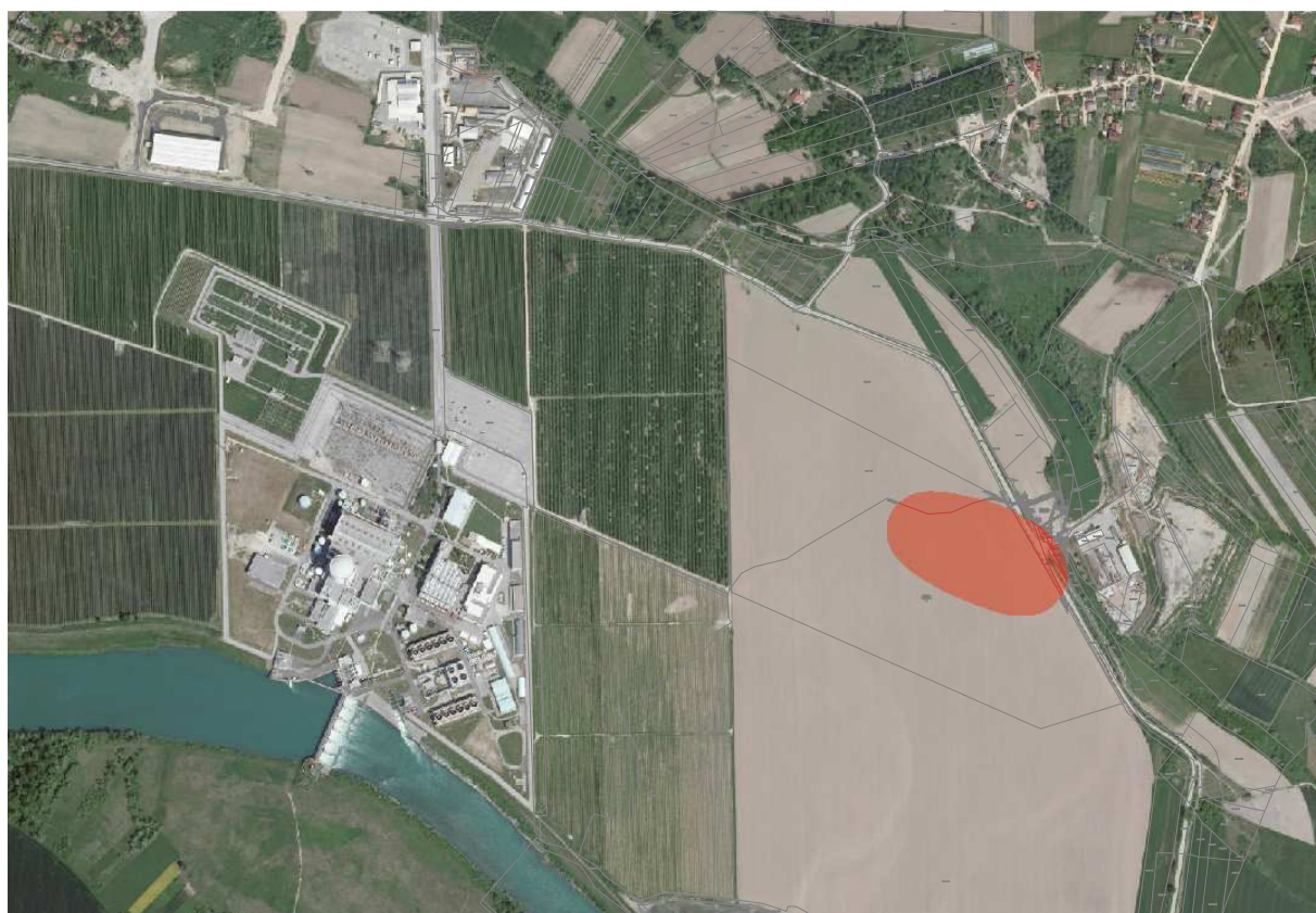
Figure 2: Impact area during construction of embankment
